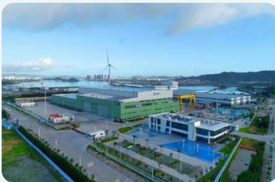
Shantou Smart Energy Demonstration Project
