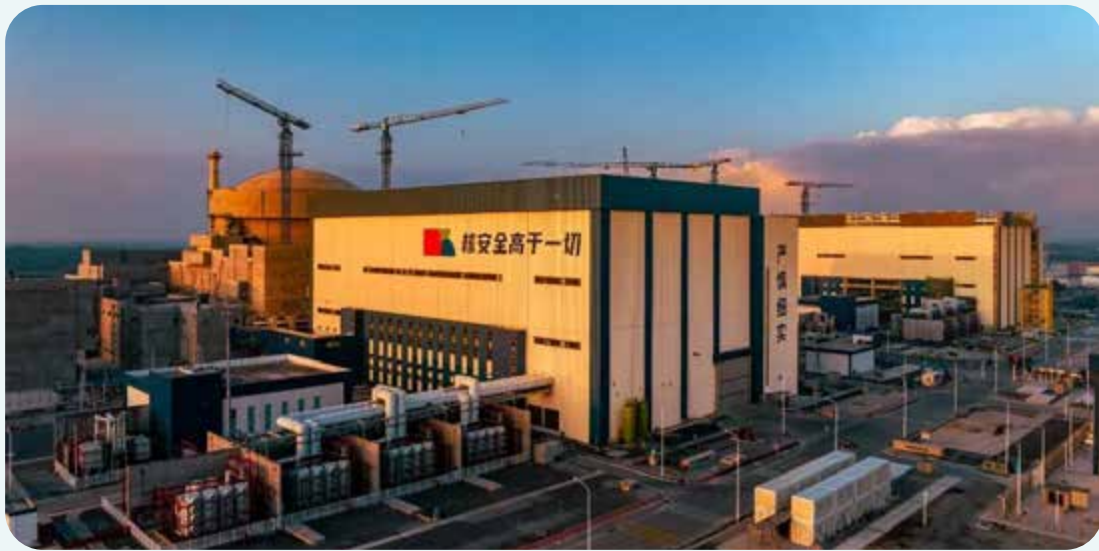
"Hualong No. 1" Fangchenggang Unit 3 was connected to the grid
