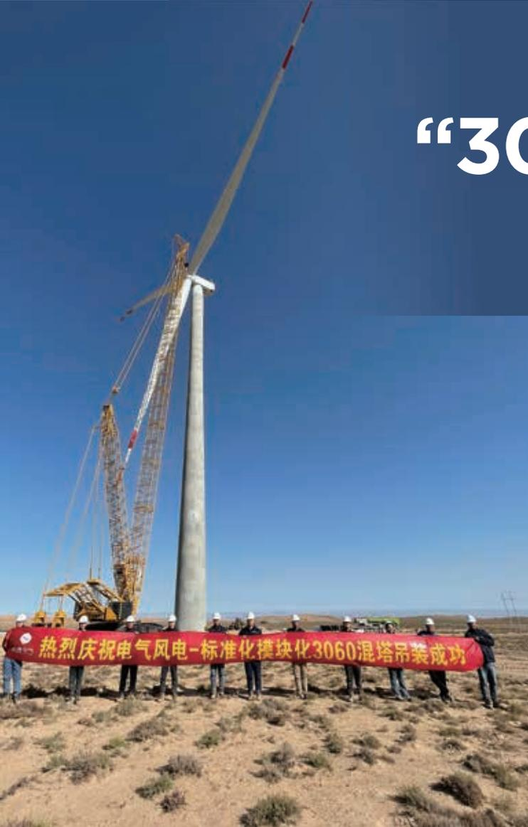
in regions with a low wind speed and high wind shear value due to its high rigidity, security, stability and low raw material cost. The “3060 hybrid tower” solution designed is customized by Shanghai Electric Wind Power for the new large-capacity turbine under all circumstances with high profitability.
