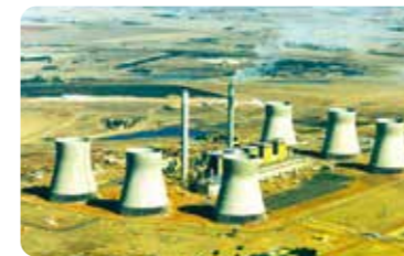
Kendal South Africa Indirect Dry Cooling System 6X690 MW
