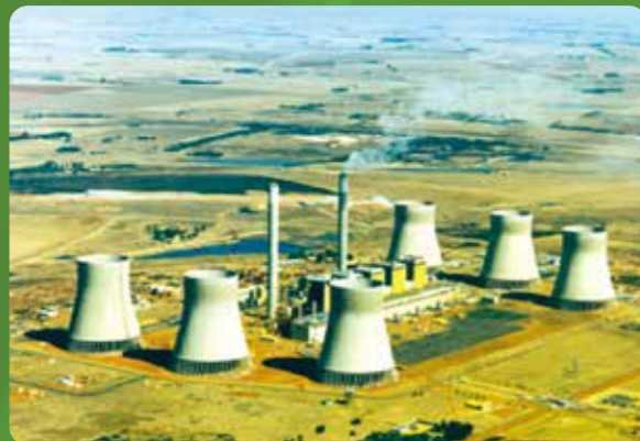
Kendal South Africa Indirect Dry Cooling System 6X690 MW
