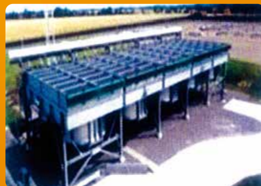
Mechanical Draft Cooling System
