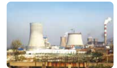
Shaanxi Qinling IDCT 2x600MW
