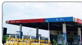
Hydrogen refuel station
