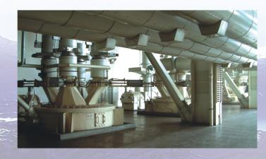
The capacity of mill is decided by primary air, and it is no direct relationship with the speed of coal feeder. The coal feeding quantity coming into the mill is controlled base on the coal level in the mill. A certain quantity of coal must be kept in the mill so as to reach its optimum pulverizing effect. For this purpose, the coal level inside the mill must be measured all the time.
