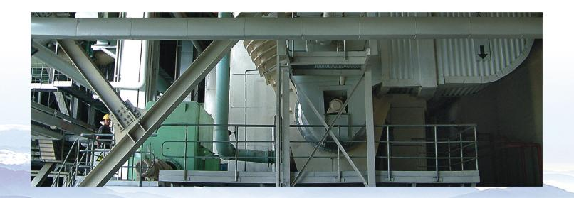
The raw coal unloaded from the bunker through the coal feeder equipped with automatic speed control drops into coal mixer. After pre-drying by by-pass air, the coal is pushed into mill tube by a spiral conveyer and then it is pulverized by means of moving balls in the rotating tube.
